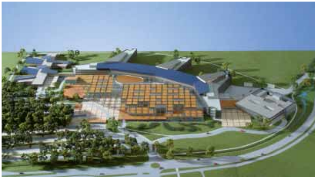
Figure 1 View of Deventer Hospital
