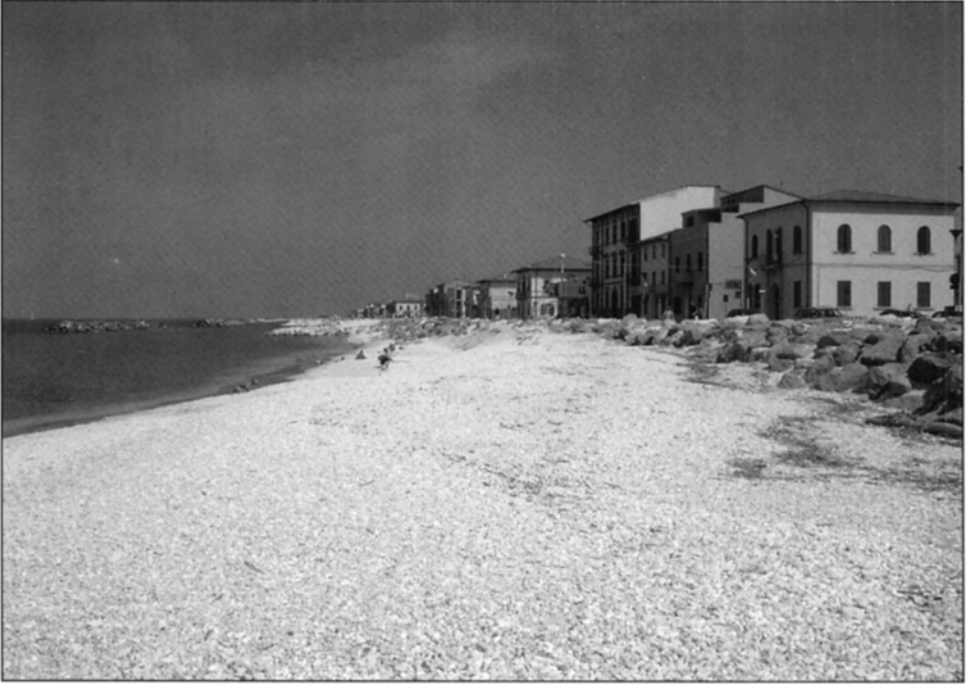
FIG. 4—The marble beach in the more southerly of the two beach compartments at Pisa 1 in May 2006. The beach near the marble groin in the background narrowed after the fill, and gravel is thrown onto the road during storms, requiring use of earth-moving equipment to return overwashed sediment to the beach. (Photograph by Karl F. Nordstrom)
