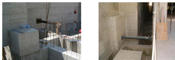
Figure 11 View of a steel spacer and the corresponding spring-damper, before and after the installation of the latter
