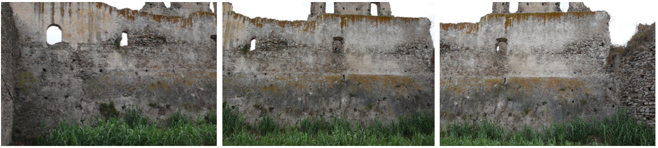
Figure 6. Photographic survey of the elevations
