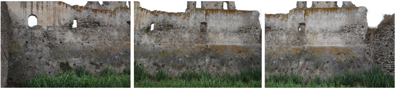
Figure 6. Photographic survey of the elevations
