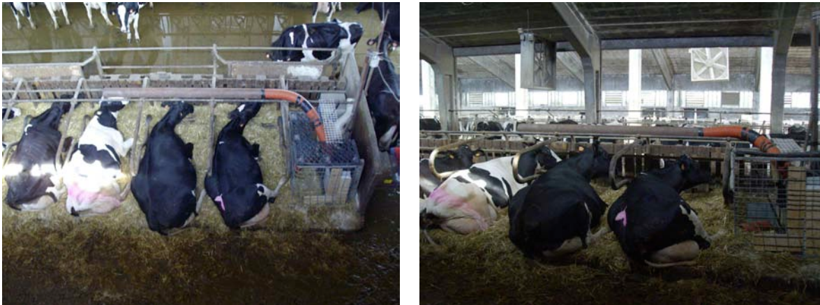
Figure 5. The experimental localized air cooling system applied in three cubicles.
