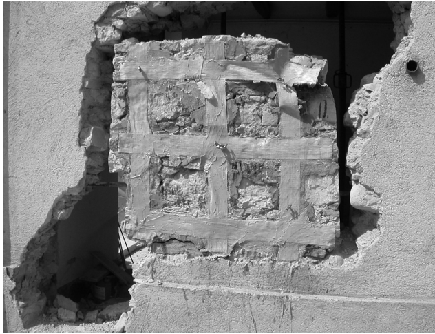
Figure 19 A panel retrofitted with GFRP sheets
