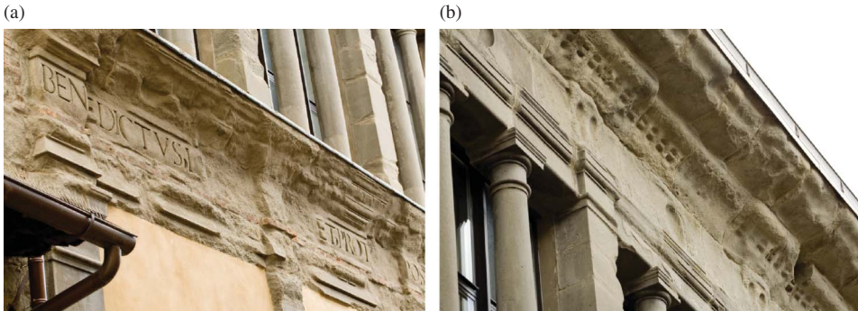
Figure 8a, b. Details of the Palace after restoration (color figure available online).
