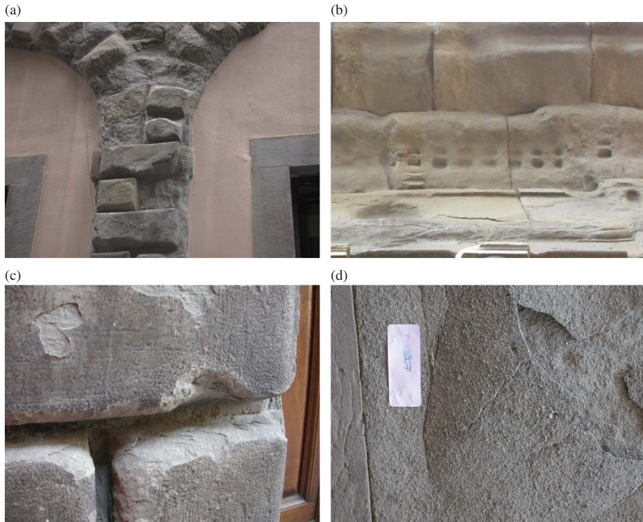
Figure 3. Different decay phenomena at variable scales: erosion, scaling (a), decohesion and dissolution (b), flaking and scaling (c), swelling (d) (color figure available online).
