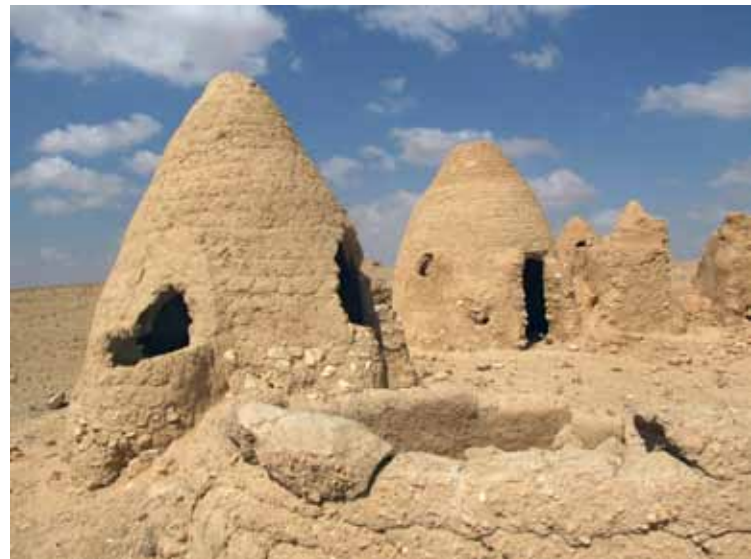
Fig. 19: Dewar technique or cob, is composed of earthen rows of mud in Hama region. Fig. 20: Thickness of dome base is variable from place to another in South Aleppo.
