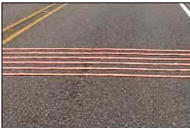
FIGURE 5 Raised transverse in-lane rumble strips.
