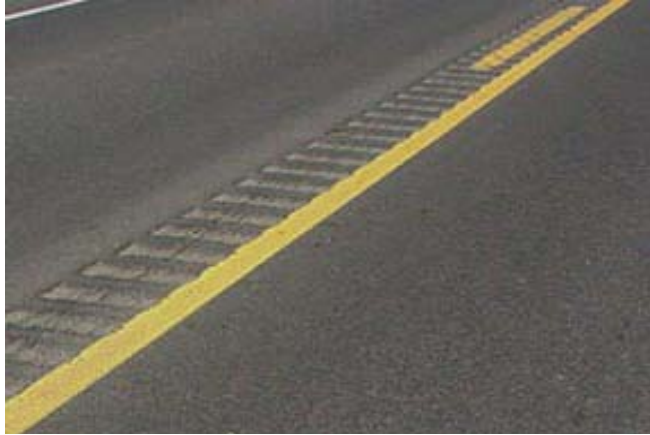
FIGURE 4 Centerline milled rumble strips.
