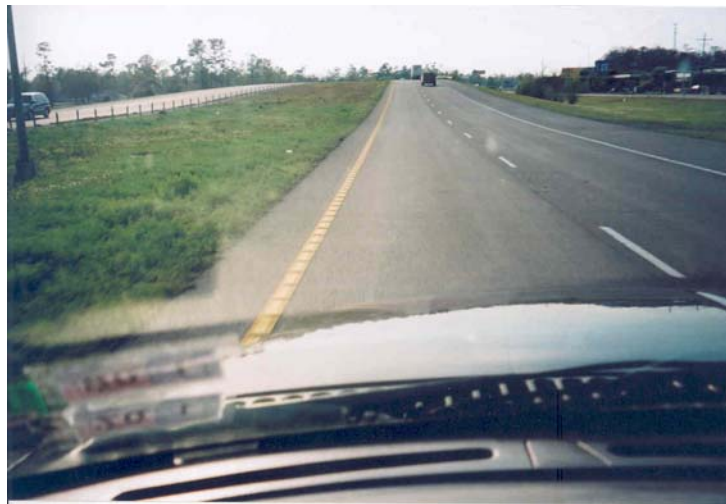
FIGURE 3 Permanent raised pavement markings.
