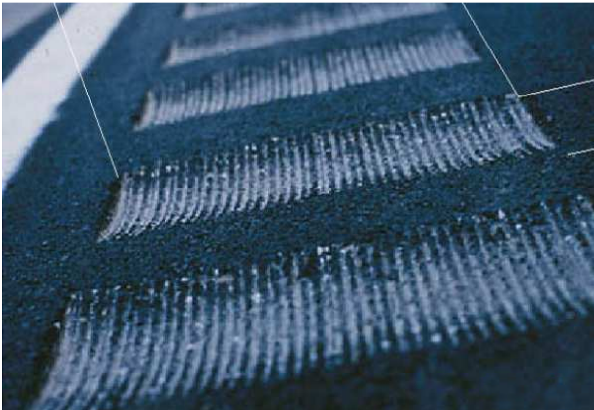
Figure 19: shoulder rumble strips [23]
