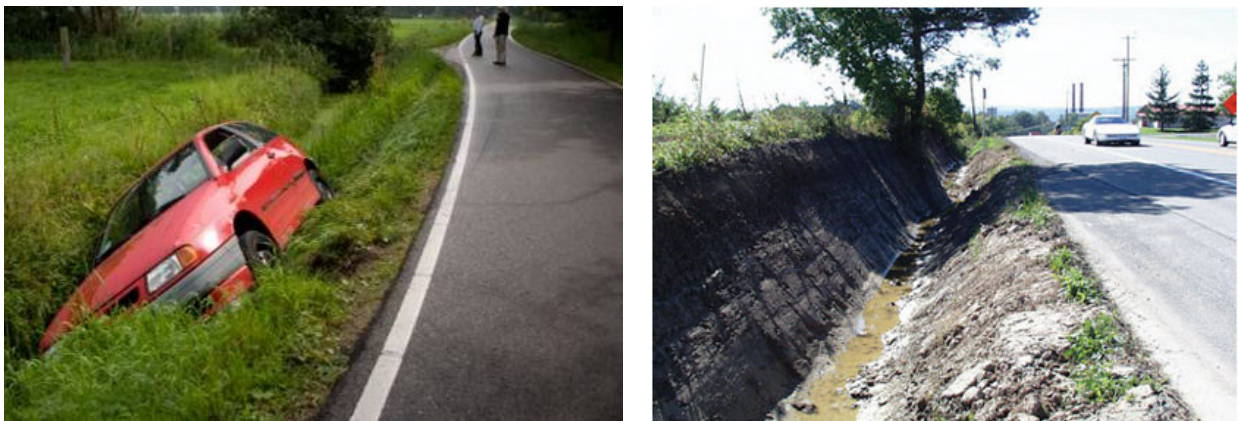
Figure 13: Examples for hazardous roadside ditches (Source: [B.8])
