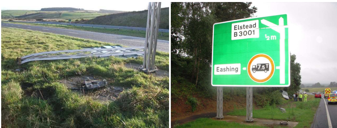
Figure 39: “passively safe” sign support after being hit by a passenger car [57]
