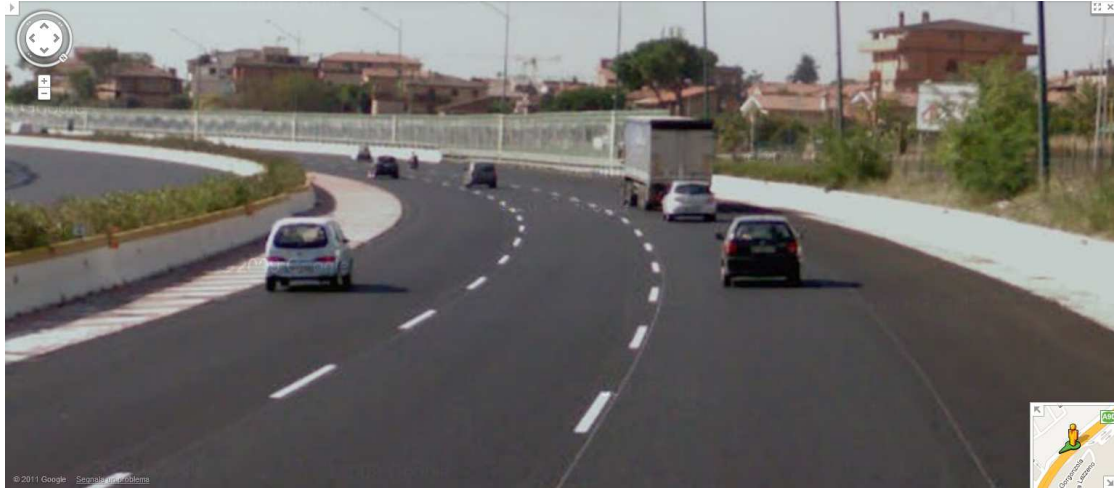
Figure 28. Raised rumble strips used in the left shoulder in the Rome Beltway.
