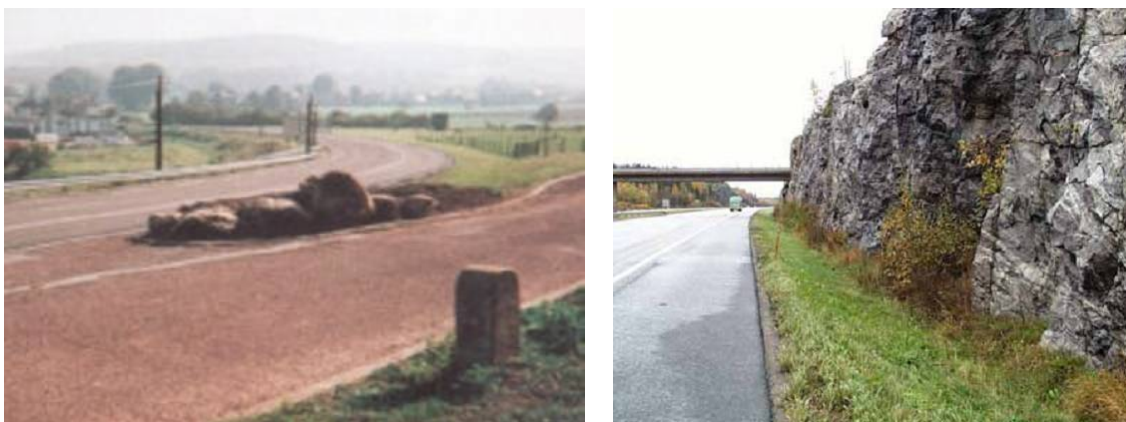
Figure 10: Examples for hazardous boulders (left) and rocks (right) on the roadside (Source: [A.2] and [A.3])
