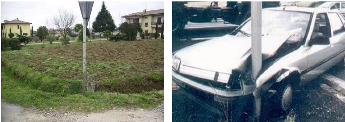
Figure 7: Examples for hazardous sign poles (Source: [A.3])
