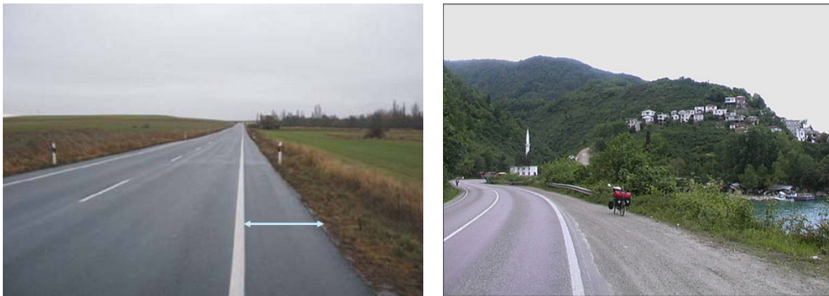
Figure 21: Examples of a hard (left) and soft shoulder (right) (Source: [A.4])
