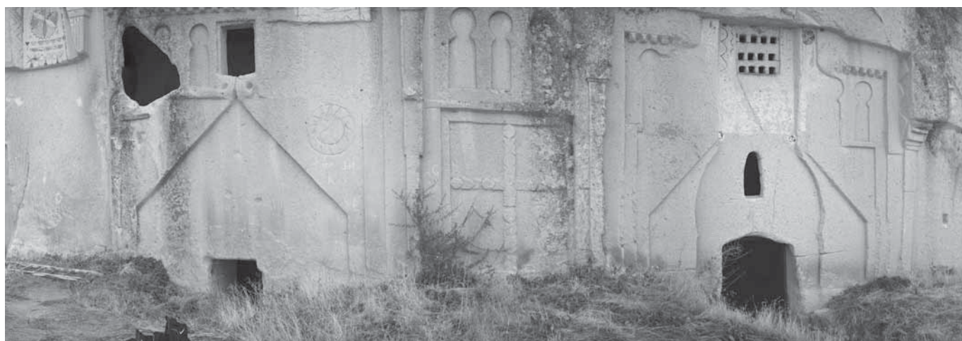
Fig.5: the east side
