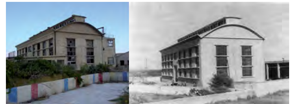
Fig. 8. The old power factory (Programming and Documentation office)
