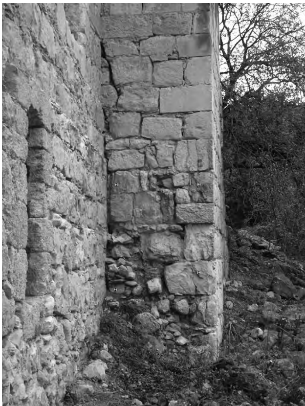
Fig 21 - Guest house: detail of hanging between the nucleus and the enlargement.
