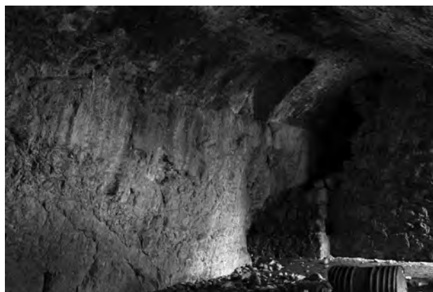
Fig 16 - Guest house: ground floor, detail of the rock wall with the vault.
