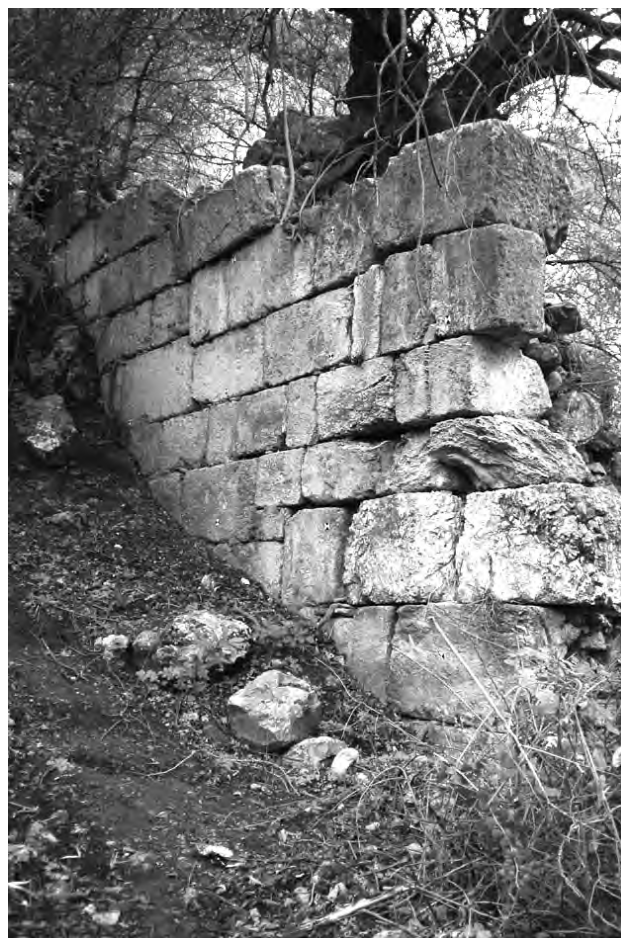
Fig 24 - View and design of the east side of the dam.
