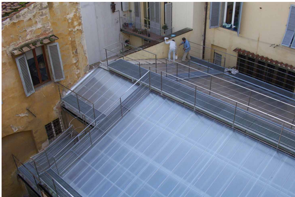
Figure 14. The new skylight: external view.
