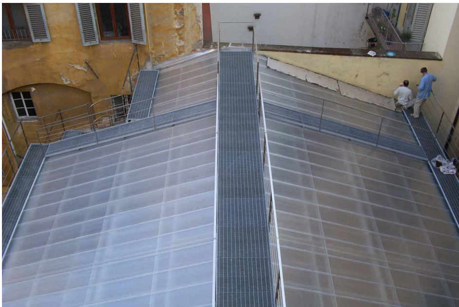
Figure 12. The existing skylight: external view.
