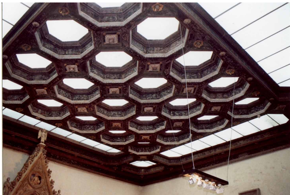
Figure 15. The existing skylight: internal view.
