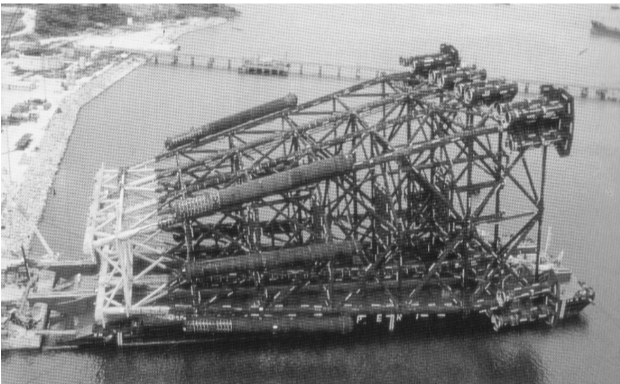
Fig. 1: Vega A, Steel jacket platform.
