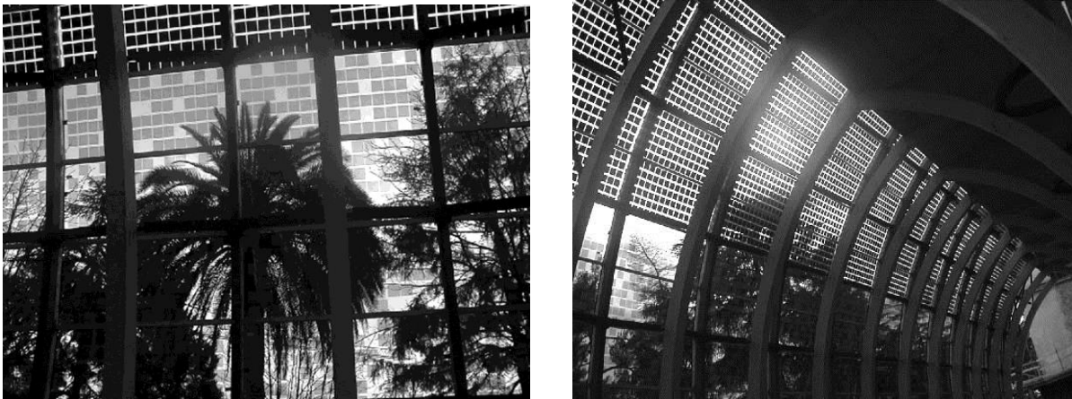
Figure 3: The PV plant integration in the greenhouse
