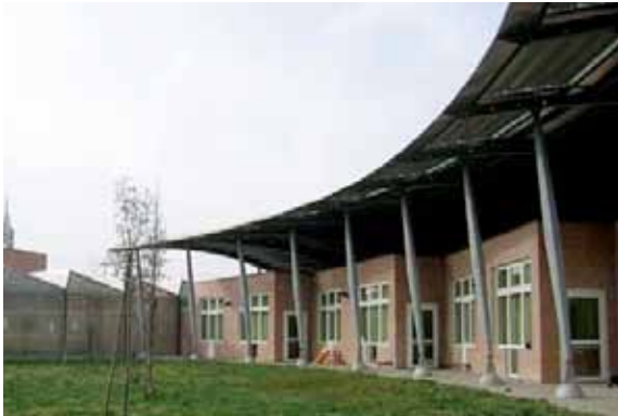
Pic. 01 - Kindergarten school in Ponzano. The wall insulation helps to increase the well-being indoor in order to reduce noise and to save on energy costs.
