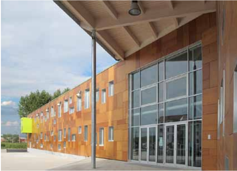
Pic. 60- Piobesi Torinese Elementary School, Archiloco Studio Associato the use of photovoltaic and solar Thermic panels, geothermic and green roof, natural ventilation chimneys low emission glass, permits the school to have a usage of 3,6 kwh/mc/year.
