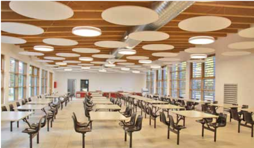
Pic. 02 - Elementary school canteen "Cesare Battisti", Fiume Veneto Pordenone. There are acoustic circular elements with a diameter between 1.2m and 1.85m, detached from the ceiling in order to optimize the sound absorption on both faces of the elements.
