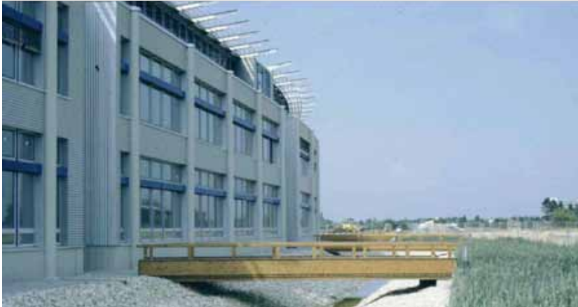
Pic. 08 - Bonn-Rhein-Sieg University. The rainwater coming from the roof is collected in a reservoir (the gap) at the entrance of the school building.
