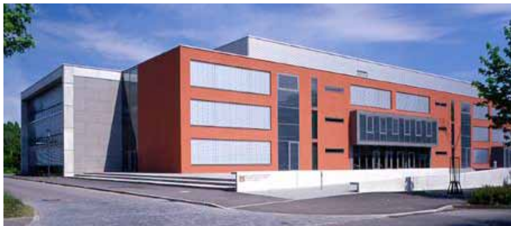
Pic. 07 - Gebhard Muller Discript school centro Biberach. In the school there is a 1.5-m3 tank for collecting rainwater.
