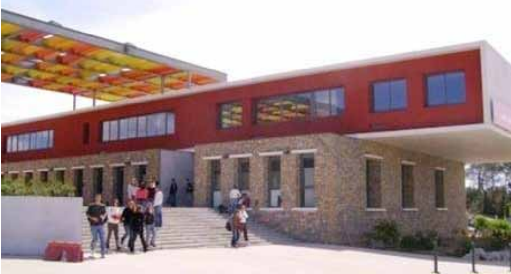
Pic. 14 - School St Clément de Rivière, France
