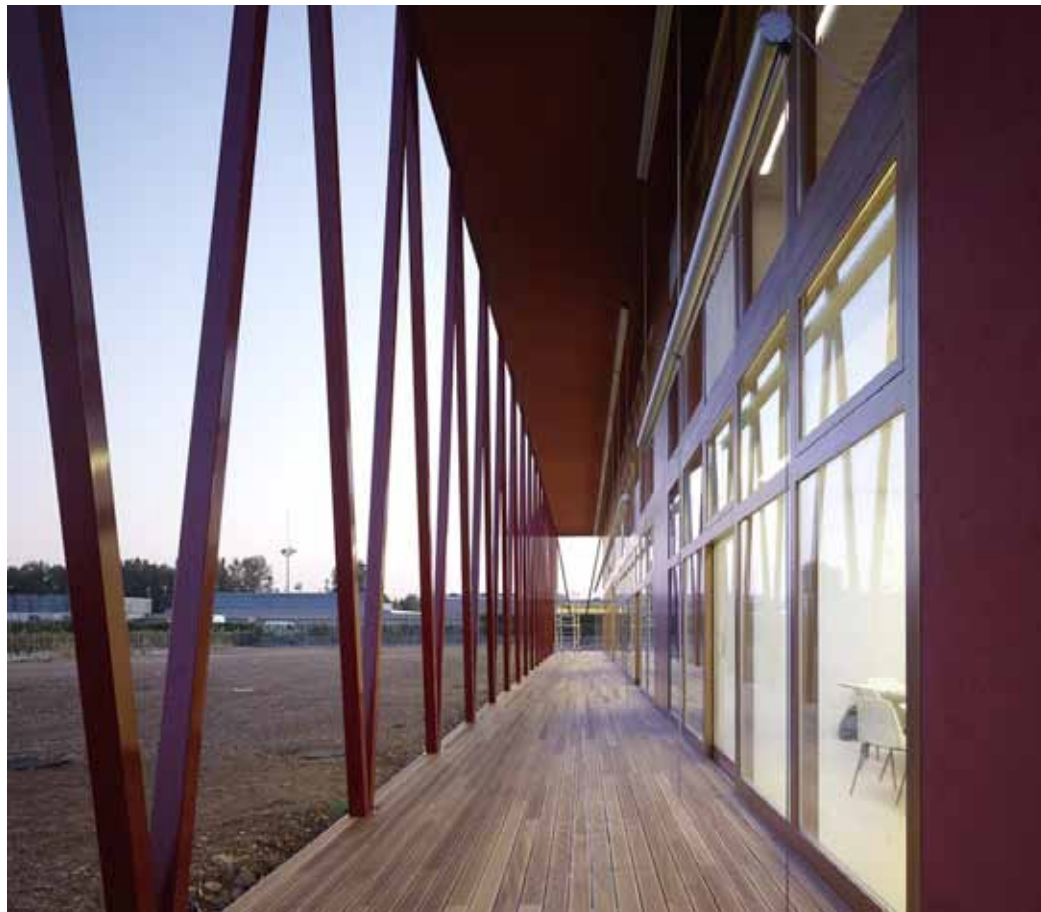
Pic. 59- Ponzano- Treviso Elementary school
