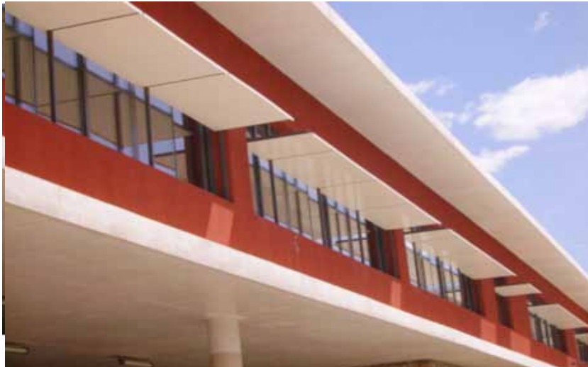
Pic. 15 - The classes oriented to the south are protected from direct sunlight by metal shielding devices (light shelves) that reflect directed light at the white ceiling of the classrooms.
