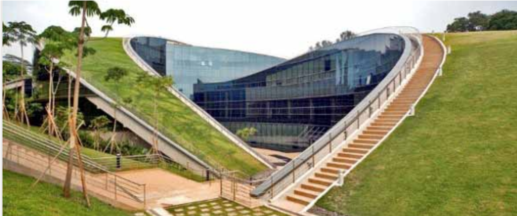
Pic. 23 - The Singapore art school is a building which hosts the Design and Media school and the Nanyang Technological University. The two "hills" with stairs are accessible to students who can enjoy in complete freedom their break moments. Besides establishing an active relation with the surroundings, the natural ceiling functions as insulator and air purifying.
