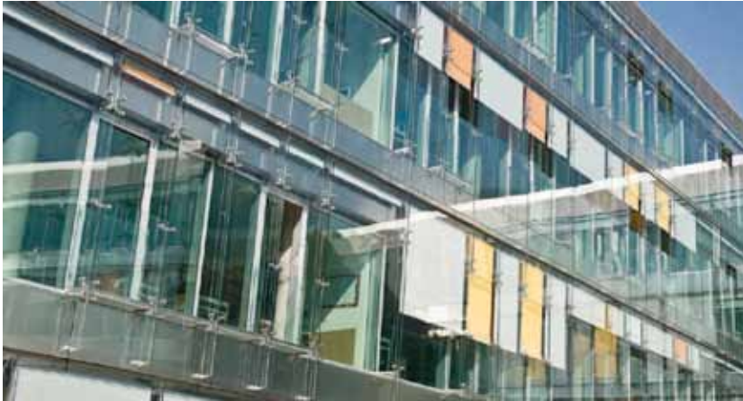
Pic. 33 - Secondary School "Giovanni Pascoli", Bolzano, Project: arch. Ranzani
