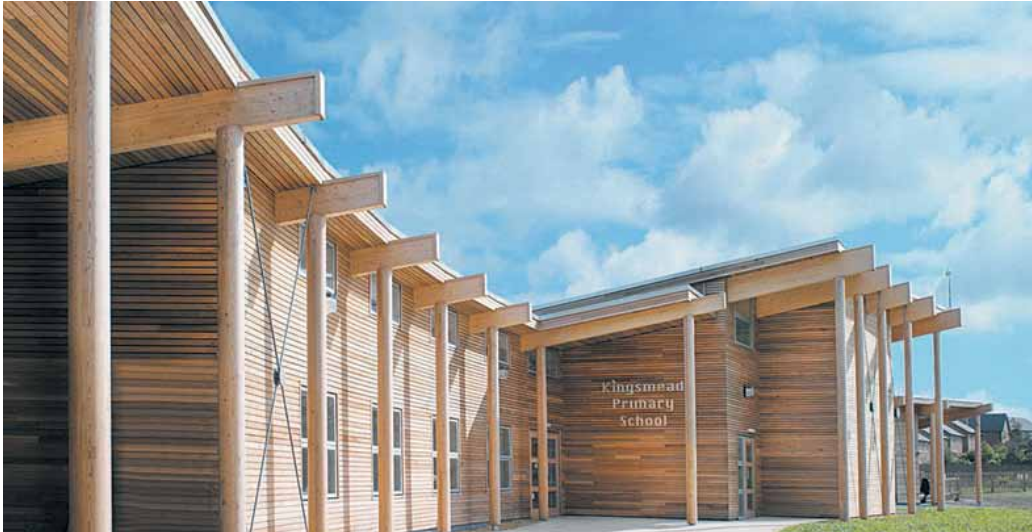
Pic. 11 - Kingsmead Primary School, North England
