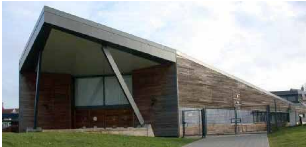
Pic. 05 - Elementary school "Notley Green"
