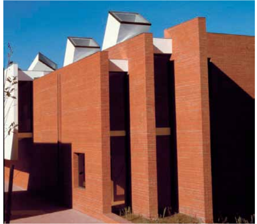
Pic 38 - Primary School Belas
