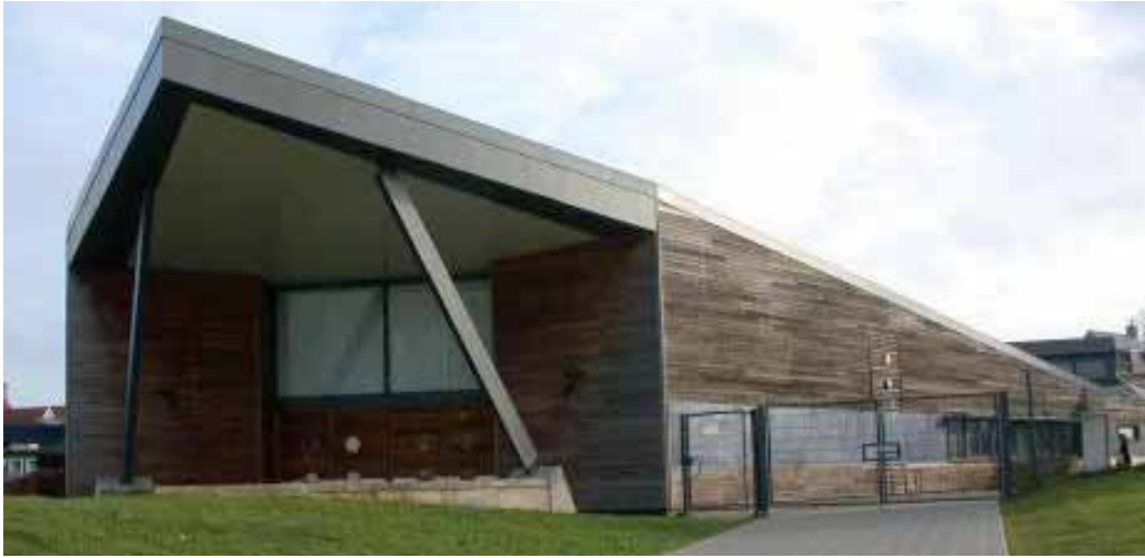
Pic. 05 - Elementary school "Notley Green"
