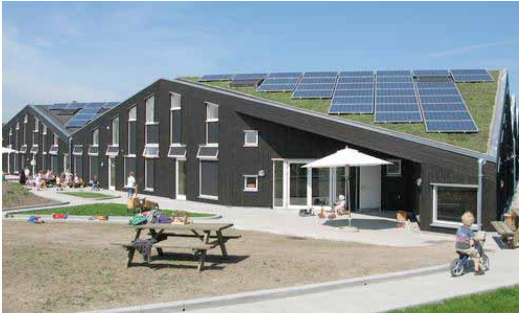
Pic. 30 - The new triangular school building by architects Christensen&Co, Horsholm, north of Copenhagen, Denmark, not only produces more energy than it needs, but offers to the children, in spite of its compact shape, perfect natural lighting conditions.
