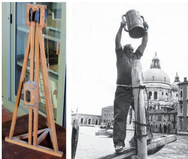
Figure 1. Pile driver model, owned by the GESAAF, and a present-day hand operated pile driver in Venice.
