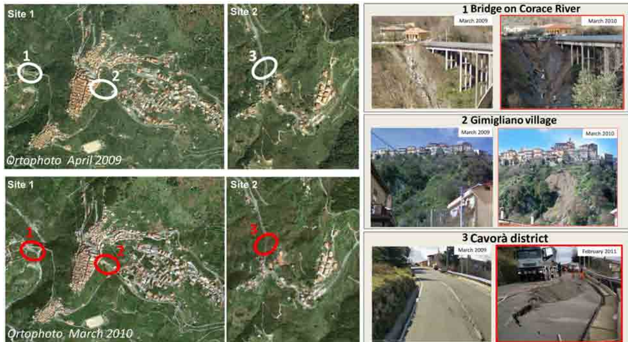
Figure 3. Location and date of recent landslide occurrences in Gimigliano area (1) landslide on the scarp along Corace river, damaging Corace bridge pylons; (2) landslide on metamorphic rocks slope, threatening Gimigliano Superiore buildings; (3) landslide in Cavorà district.
