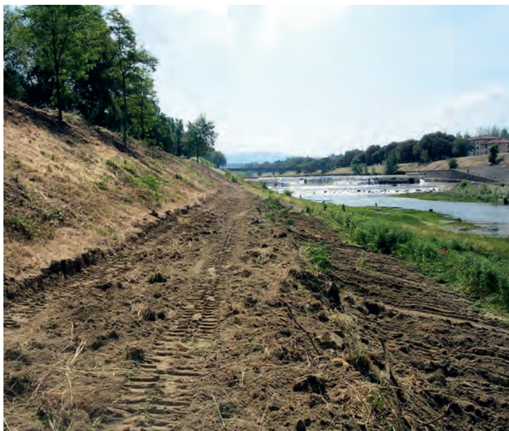
Work in progress: June 2005
