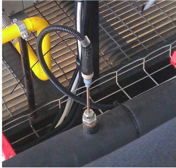
Figure 56 - PT100 temperature sensor
