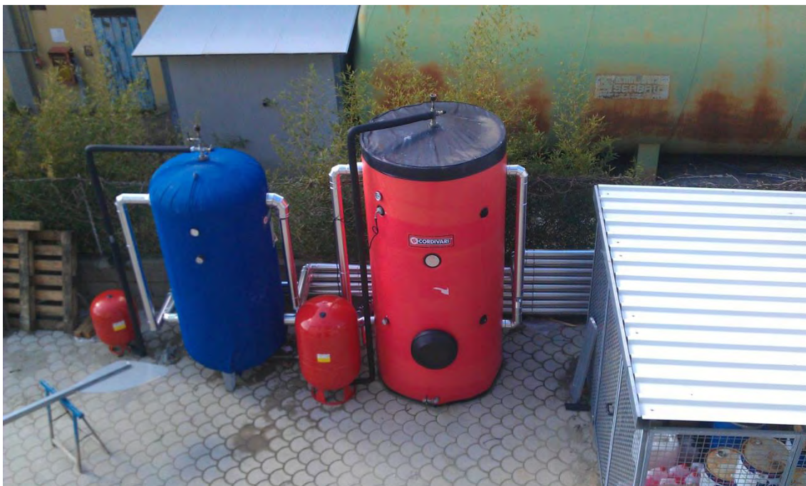
Figure 39 - Thermal storages: "cold" (blue) and "hot" (red)
