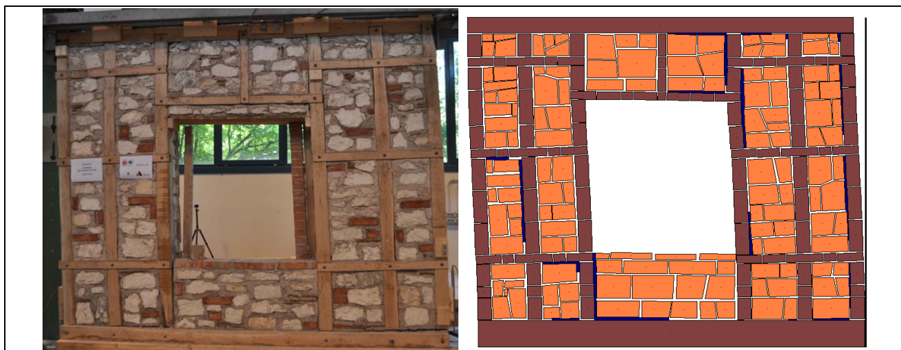
Figure 9. Ultimate deformed shape and cracking pattern. Comparison between experimental test and numerical modelling.
