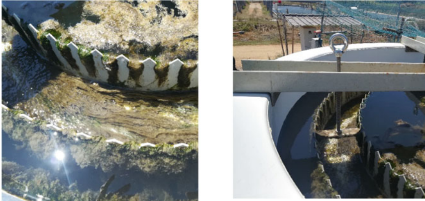
Fig. 4 Algal bloom within the weir and radial settler view without cover cap
