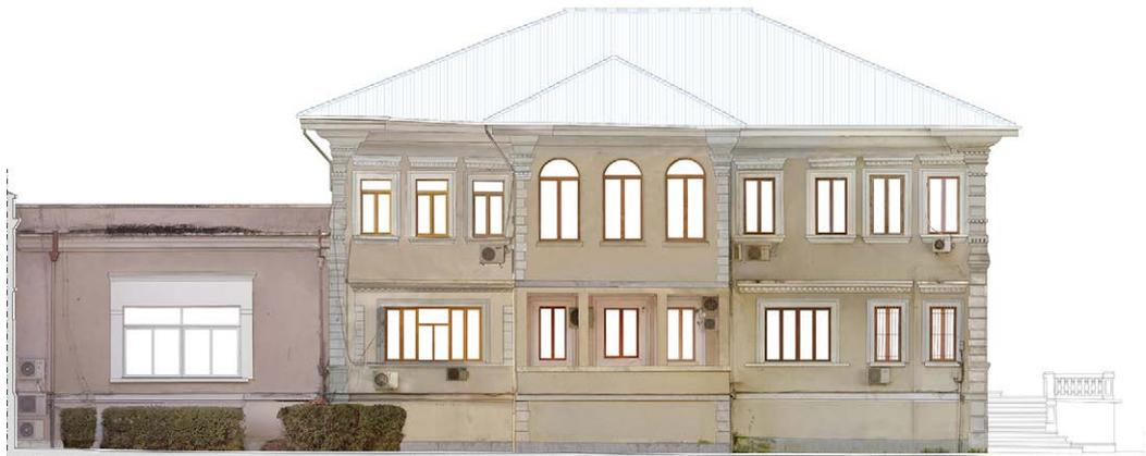
is possible to infer how the first-floor bow window was originally supported by corbels and, only later on, it was added the loggia at the lower level, a feature that currently characterizes the front.
