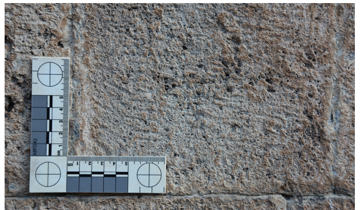
[fig. 5] Above: an overall view of the western side of the Zorats' Church (E4), and of the eastern side (E2); below: a detail of the stone dressing of the main construction phase of the Zorats' Church (YGV1)
