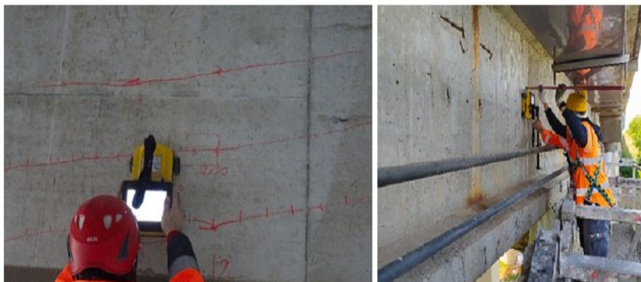
Figure 5-2: In situ execution of GPR tests.
