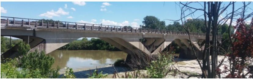
Figure 8-22: Picture of the studied bridge
