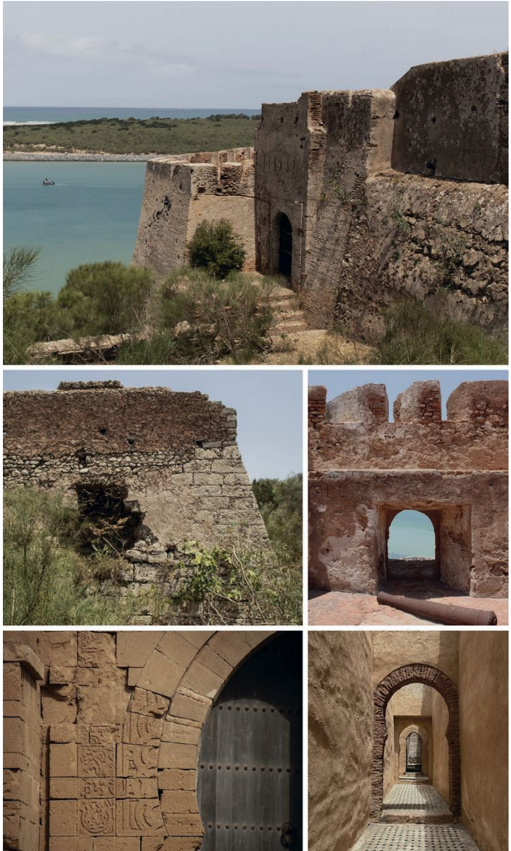
Fig. 2. Coexistence of architectural languages. The Spanish phase of the seventeenth century is recognisable in the San Guzmán bastion ( top right ), in the angular configuration of the layout ( top left ) and in the gun embrasures ( centre right ), as expressions of early modern Iberian military engineering. The Alawide phase reworks the pre-existing layout through elements of the Islamic tradition, such as the Bab Jdid portal ( bottom left ) and the interior spaces of the Governor's Palace ( bottom right ). Photographs by the authors, 2026.
