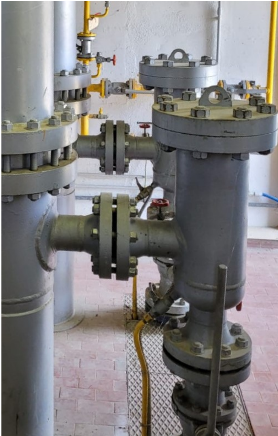
Figure 1.9: CGS filtering stage.
