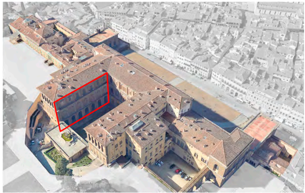
Figure 1. The Palazzo Pitti complex; The south-east facade of the courtyard is outlined in red.
