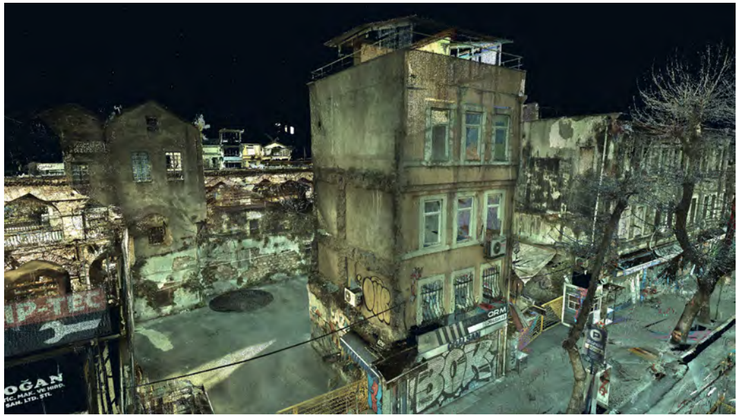
Fig. 4. Perspective view of the aligned point cloud.
