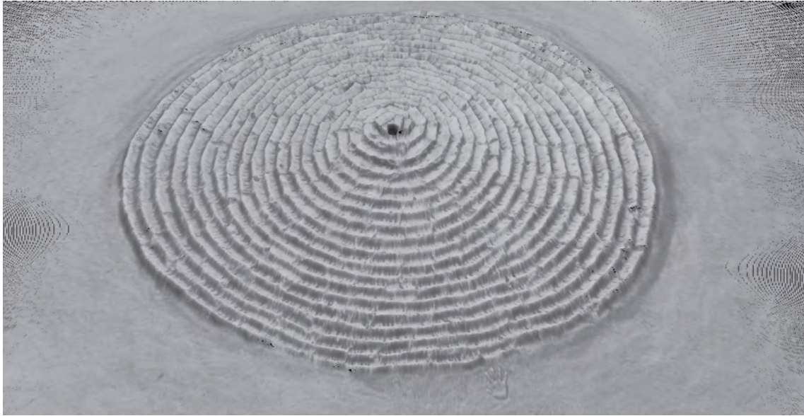
Fig. 1 The adopted solution for closing the top of the vault (inner view), the arrangement of the brick can be read easily in the 3D model (© Geomatics for Environment and Conservation of Cultural Heritage Laboratory)
