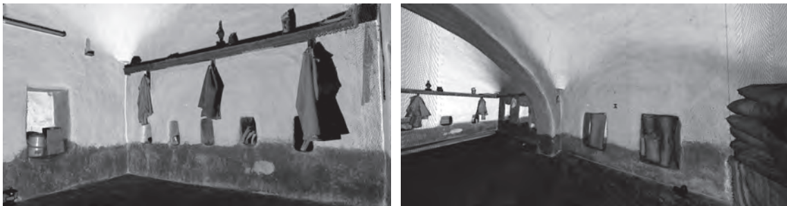
Fig. 5 Views of 3D laser scanning models: the interiors of the residences have no fixed furniture and objects are usually placed in niches. There are some very small cavities, arranged in a sequence (left), some the size of a window, or niches that rise from the floor to the height of 1–1.50m (© Geomatics for Environment and Conservation of Cultural Heritage Laboratory)
