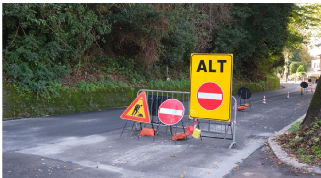
Figure 2. Visit of the worksite of Via Roma in Poggio Mirteto. Road restoration intervention due to geomorphological instability. Credits: Valeria Volpe
