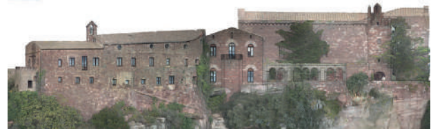
Figure 7 | Aerial images of the complex acquired by Drone DJI Mini (credits: Pietro Becherini). On the right: a general plan of the complex with the indication of the main rooms: A- church of Sant Miquel; B- Chapter room; C- South Tower; D- Cloister; E- Manor house. Below: south-east elevation with orthophoture.
