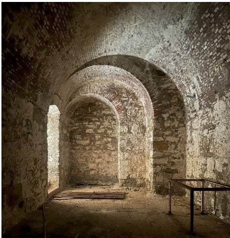
Fig.7- View of the inside towards the southern front (Marinaro, 2023).
