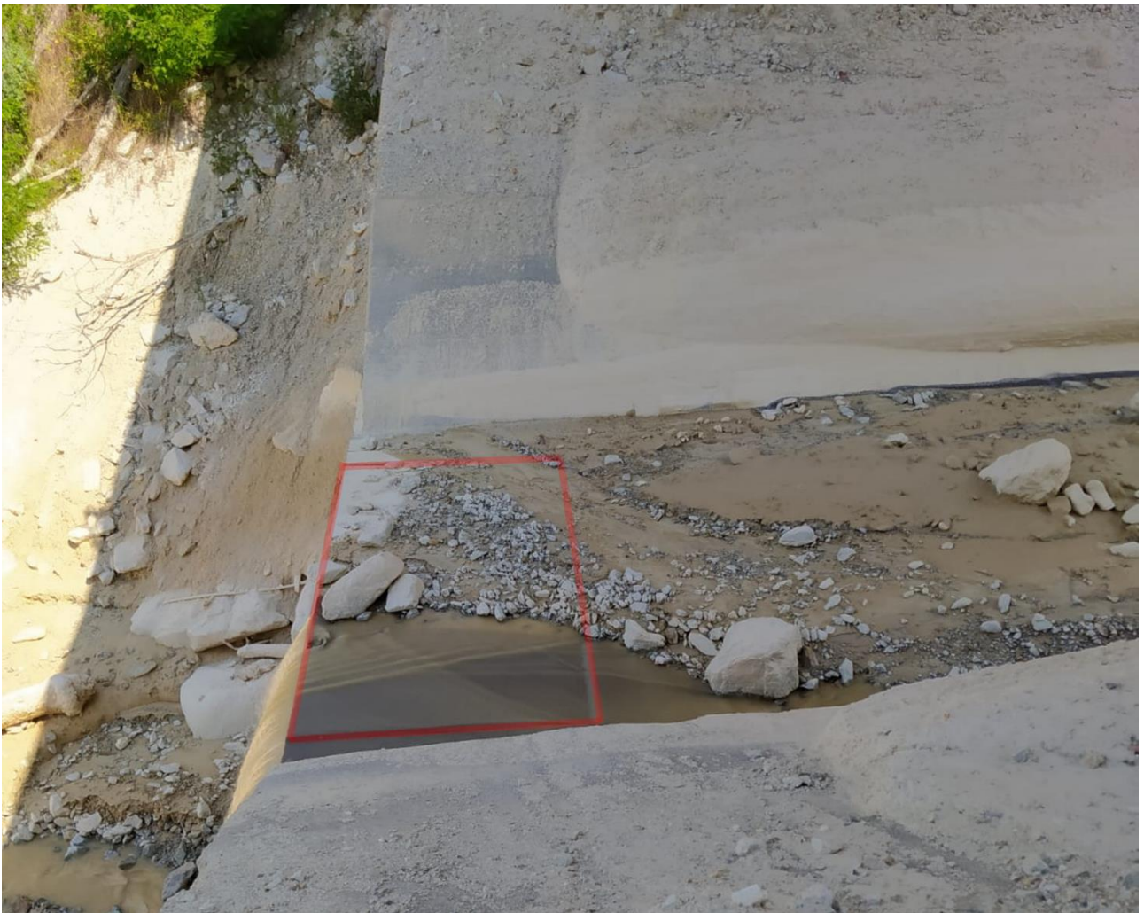
Figure 1. 23: photo of the force plate (highlighted in red) installed at Check Dam 29 at the Illgraben (Switzerland) (source: Giacomo Belli).
