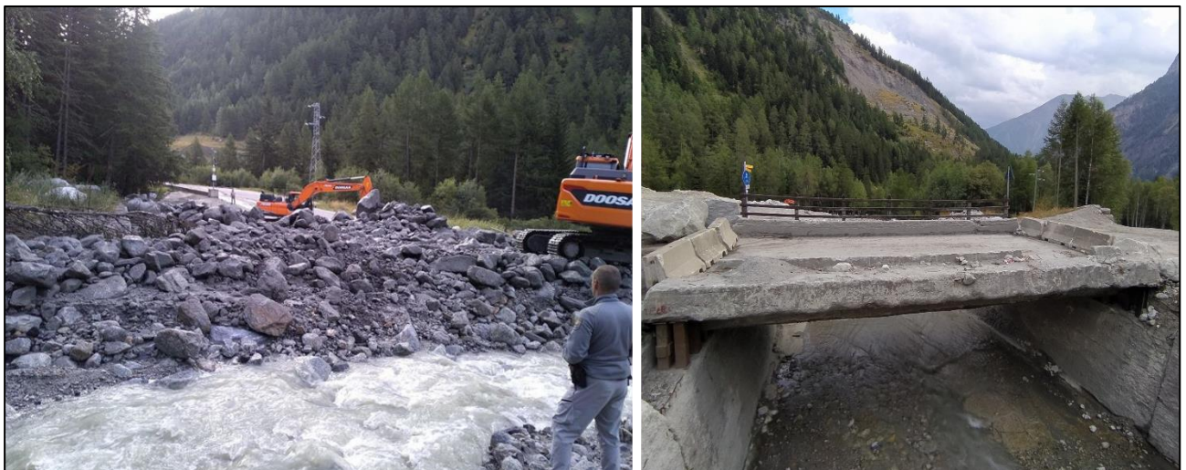
Figure 1. 12: the 5 August 2022 debris flow in the Rochefort stream (Aosta, Italy). Left: photo of the road invaded by the flow (source: Ansa.it, previously published by rainews.it). Right: photo of the road bridge destroyed by the event (source: Giacomo Belli).
