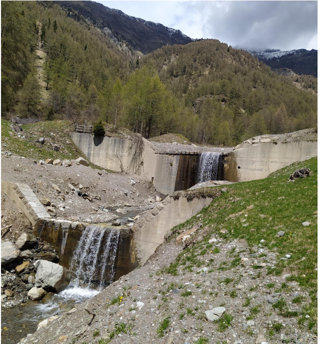
Figure 1. 16: photo of two of the several check dams realized in the 19 th century along the Gatria channel (source: Giacomo Belli).
