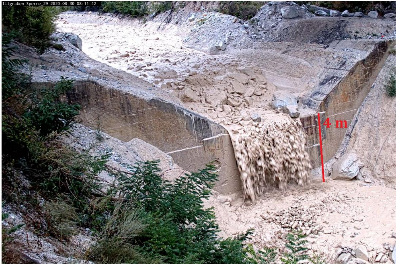
Figure 1. 3: photo (source: WSL institute of Zurich [Meyrat et al., 2021]) of a debris flow that occurred in the Illgraben catchment (Switzerland) on 20 August 2020 and flowing over a check dam realized to dampen debris-flow impact.
