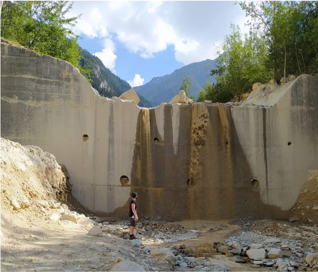
Figure 3. 5: photo of the check dam 20. With a height of ~8 m, it is the highest check dam outside the upper catchment (source: Giacomo Belli).
