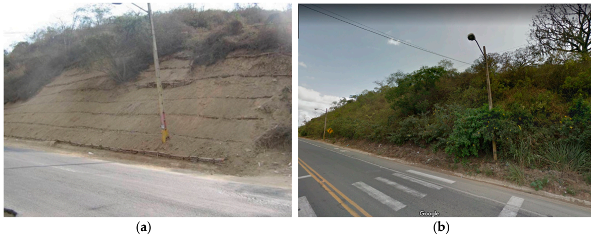
Figure 5. Soil bioengineering (SBE) construction at Jipijapa (a) after the finalization in 2008; (Petrone, 2008) (b) monitoring in 2018 (Google Streetview, 2018).
