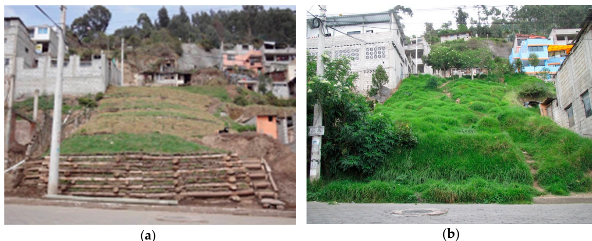
Figure 9. SBE construction in San Luis de Chillogallo in Quito (a) after the finalization in 2012; (Petroni, 2012) (b) monitoring in 2018 (Maxwald, 2018).
