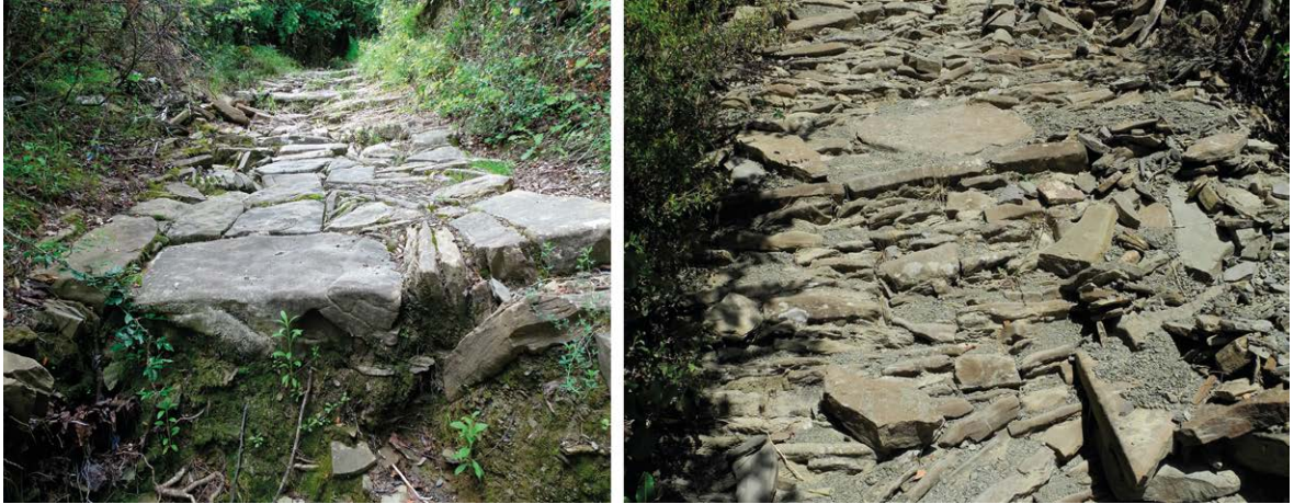
Figure 3.31 – Details of the laying of the kalldrēm .
