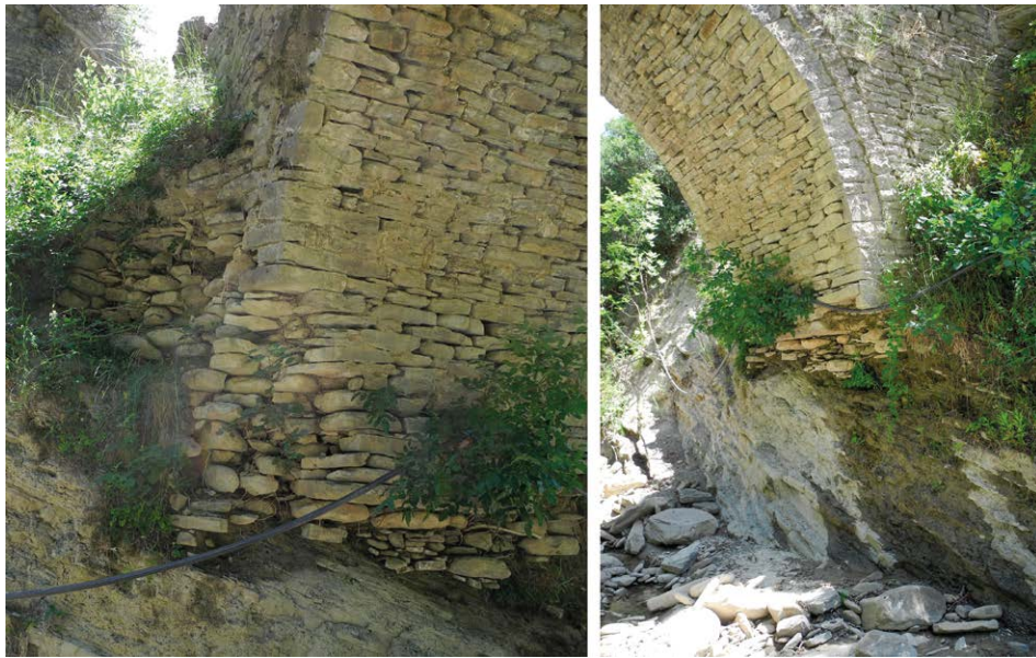
Figure 3.43 – Details of the left abutment of the Běnjě Bridge.
