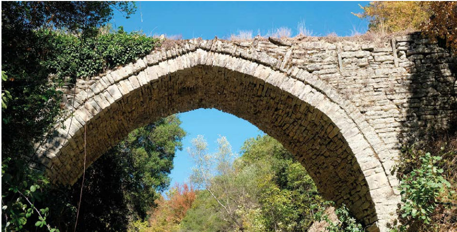
Figure 3.34 – Detail of the arch of Bënjë Bridge.
