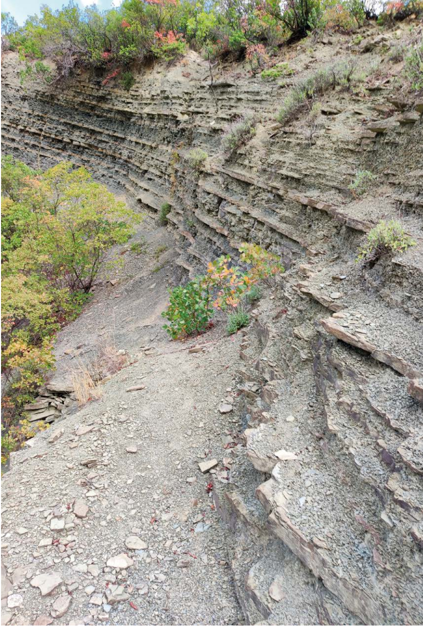
Figure 3.22 – Rock face near Bënjë Bridge.
