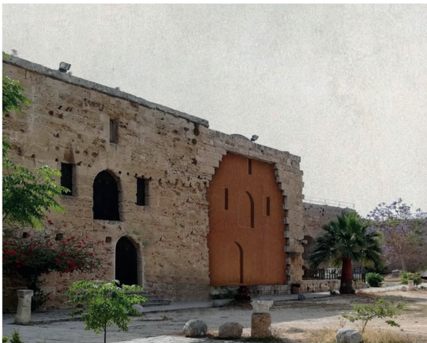
Fig. 9 - Reintegration of a missing part of the palace's façade in Corten steel (drawing E. Valletta, 2018).
