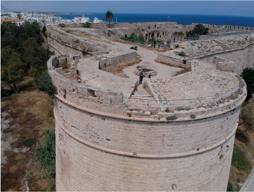
Fig. 1 – Aerial view of the Kyrenia Castle (drone photo A. Camiz, 2018).
