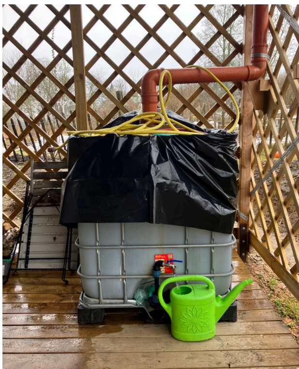
IBC tank at the farmhouse
