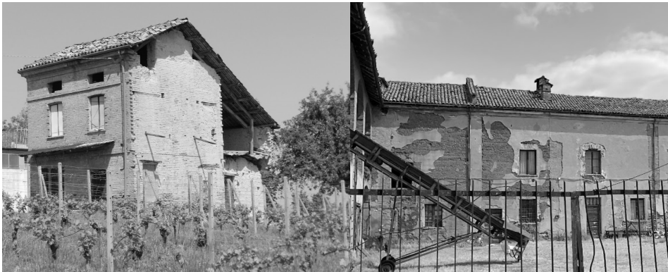
Fig. 1 and 2. Two examples of earthen buildings: to the left, an adobe building in Calosso (Asti province), to the right a rammed earth farm in Pozzolo Formigaro (Alessandria)
