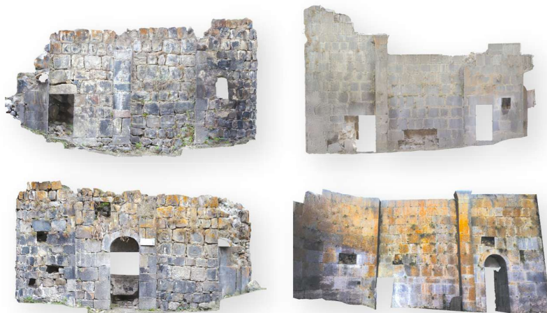
[fig. 2] A comparison between the Old Church in Yeghegis (left side) and St Sion Church of Arates (right side): above - the northern side; below - the southern side of the two churches
