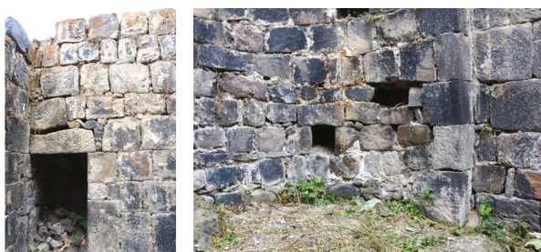
[fig. 7] On the left side, the new lintel replaced in the phase 2; on the right side, the small squared cut on the southern side
