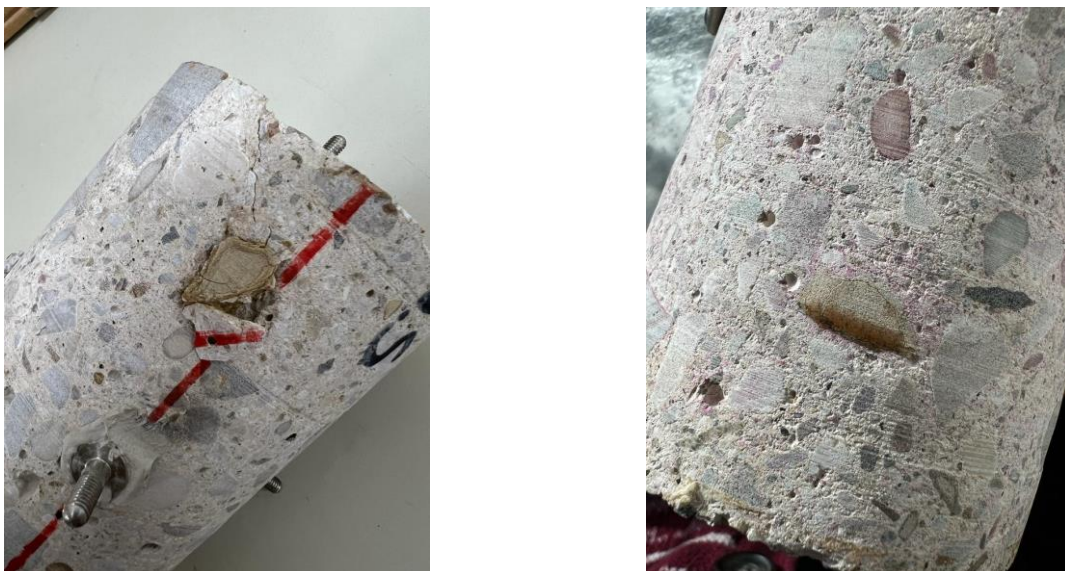
Figure 35. Concrete cores extracted from different bridges after ACPT exhibiting pop-up and gel formation.
