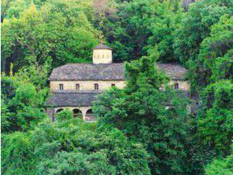
Figure I-5.3.1 View of the church almost hidden by the vegetation.
