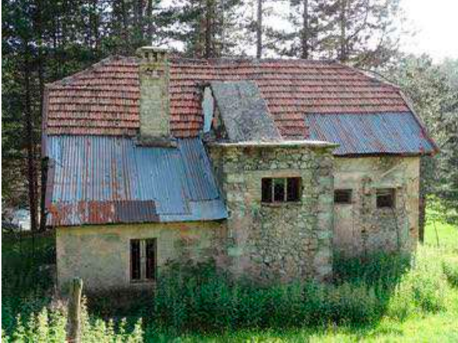
Figure II-5.8 An example of the additions and transformations that occurred over time on the rear facade of a villa.
