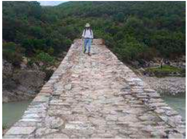
Figure I-5.1.4 – The roadway of the bridge.
