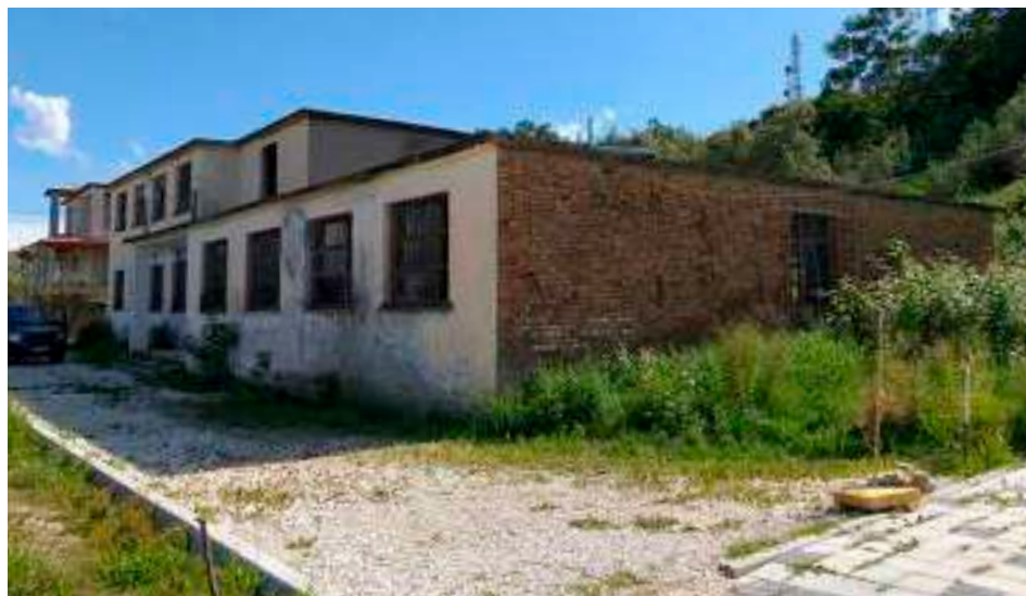
Figure III-4.4 The former village school, abandoned since 2007.
