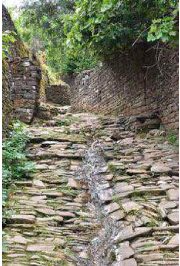
Figure I-4.3.1 – The main street of the village paved in kalldrëm and its water drainage channel in the middle.
