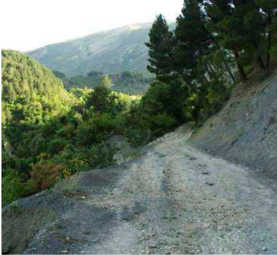
Figure I-4.3.10 The poor conditions of the road to Përmet make the life of the villagers difficult and hamper the tourism development possibilities.
