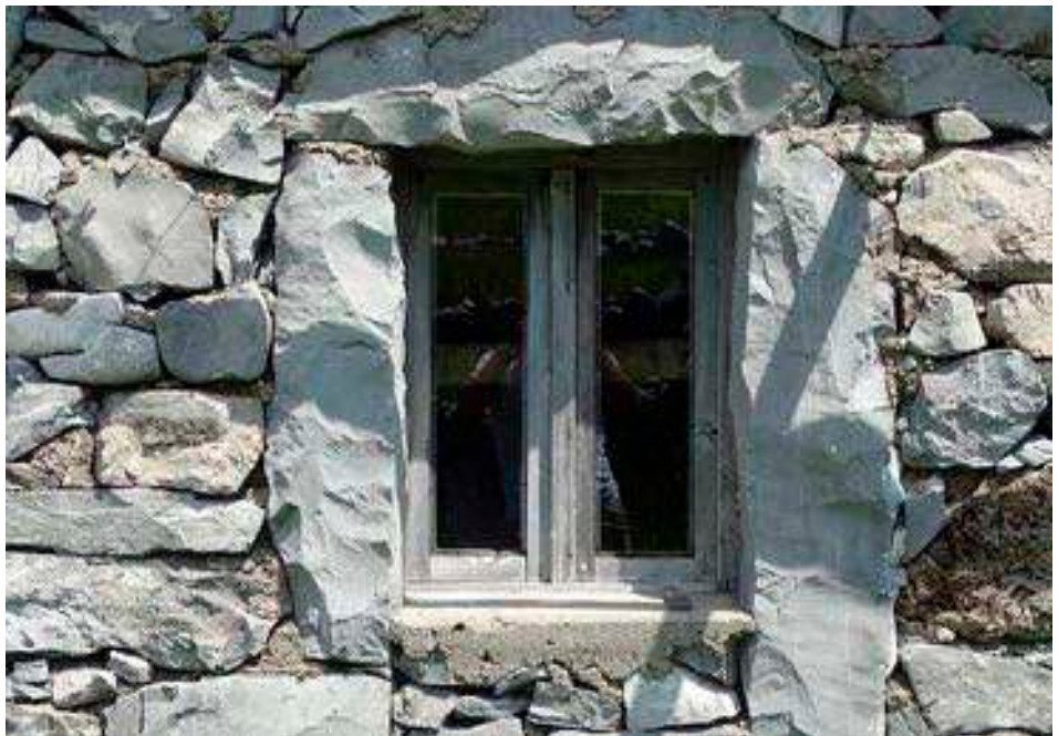
Figure II-2.9 Detail of a window with stone monolithic jambs and lintel.
