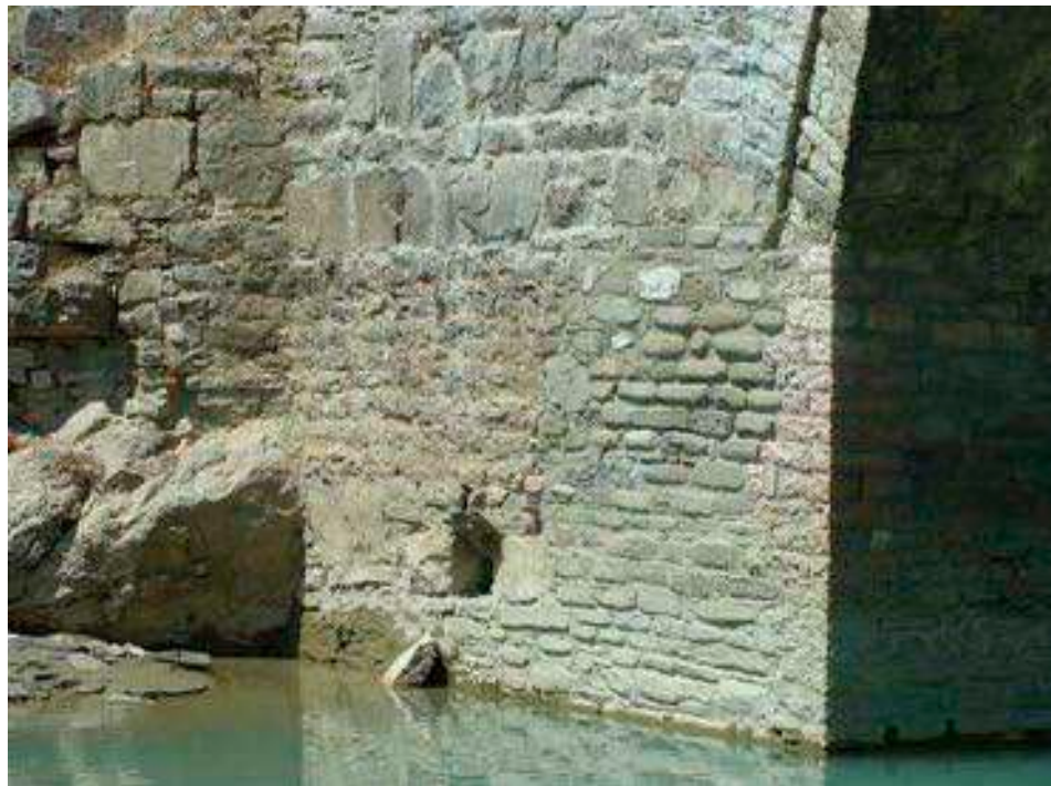
Figure I-5.1.6 – A detail of the abutment restored in 1982.
