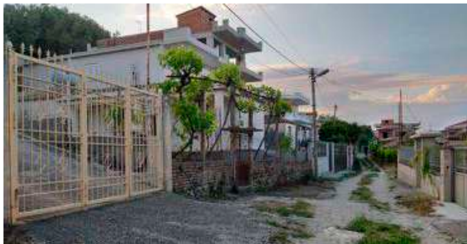
Figure III-4.8 The poor conditions of a road in the hill quarter.
