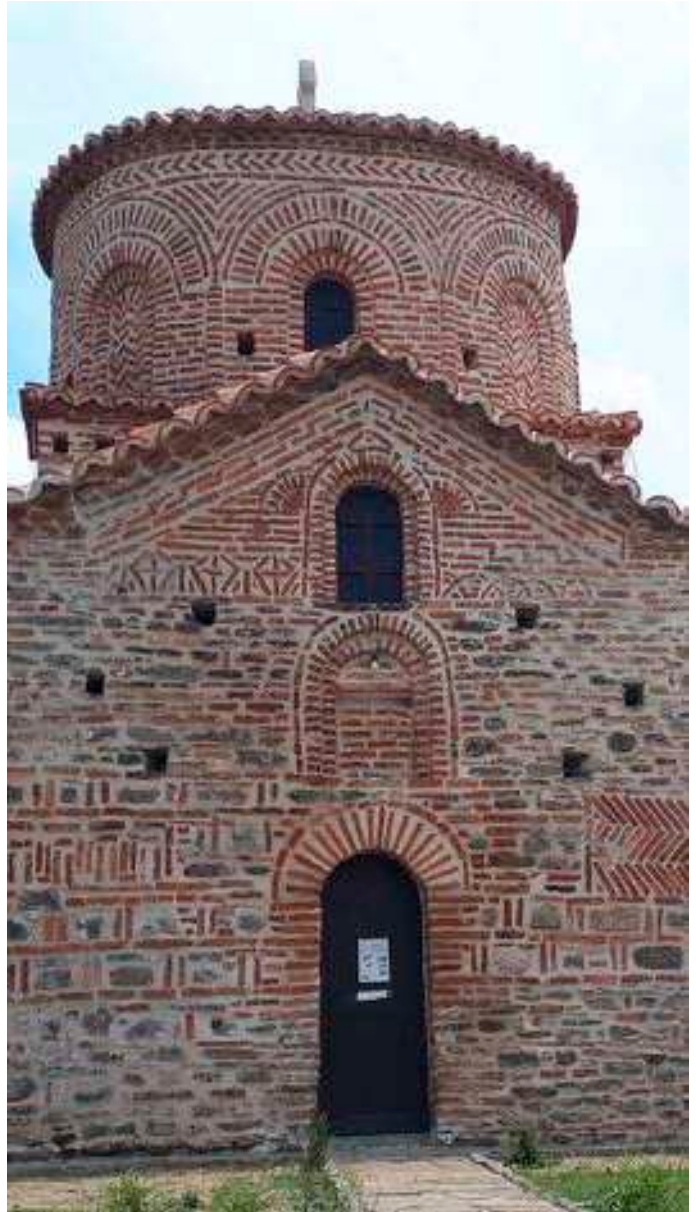
Figure I-5.2.4 – Detail of the north facade of the church with the cloisonné and other decoration techniques.
