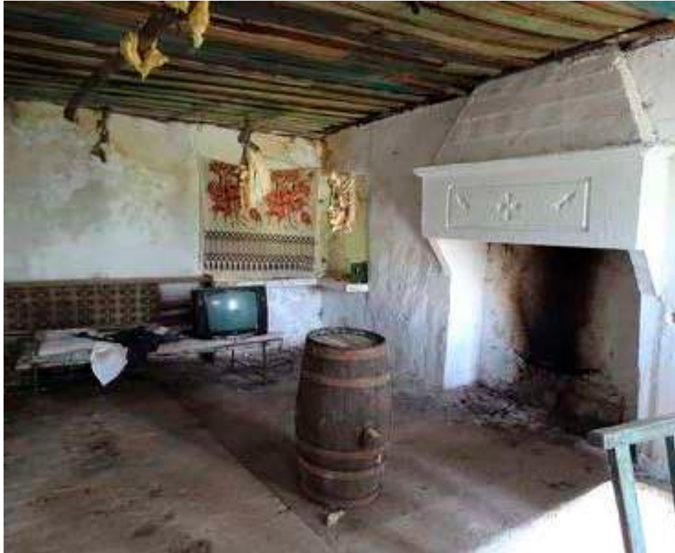
Figure II-4-11 The interior of a traditional dwelling with a wooden false ceiling and a widespread type of fireplace.
