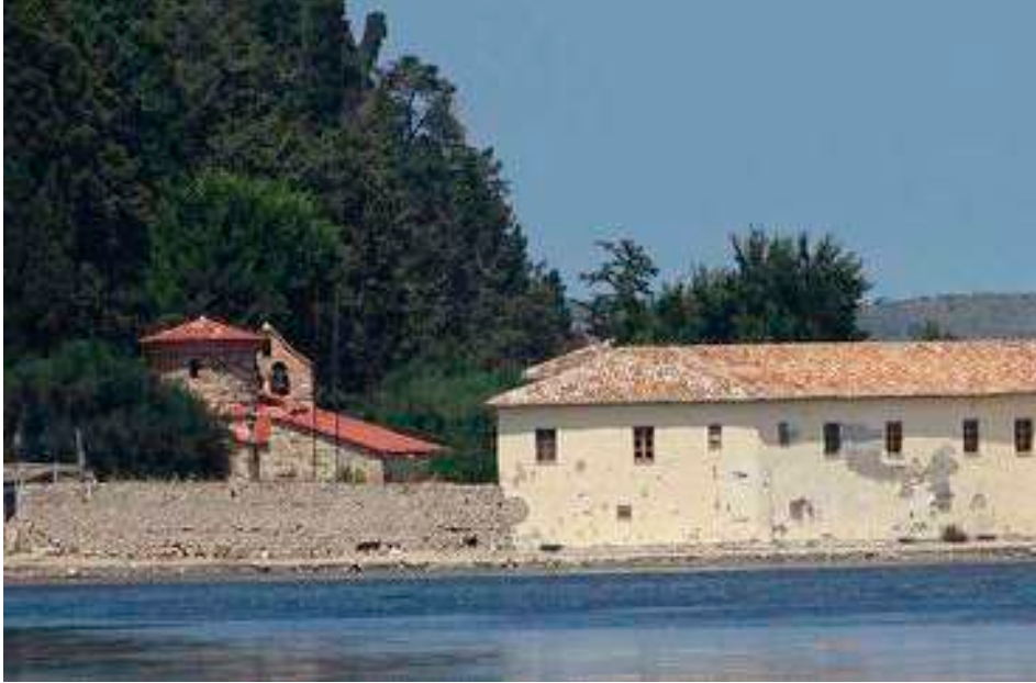
Figure III-5.9 A view that highlights the chromatic difference between the roof covering of the church and that of the lodgings.
