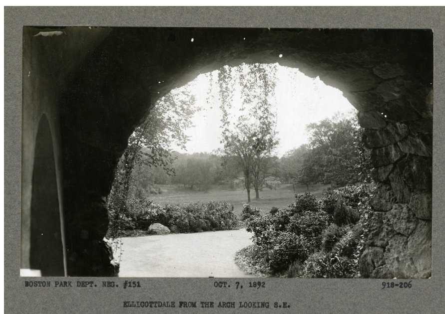
Figura 5.8: Ellicottdale Arc, Franklin park, Boston MA, USA, 1892
