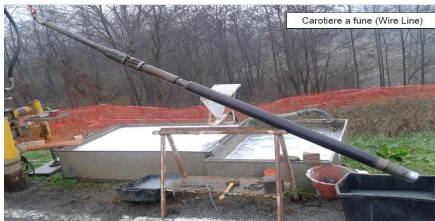
Figure 5. Wireline assembly in use (courtesy Dott. Ing. Massimo Sacchetto [12]).
