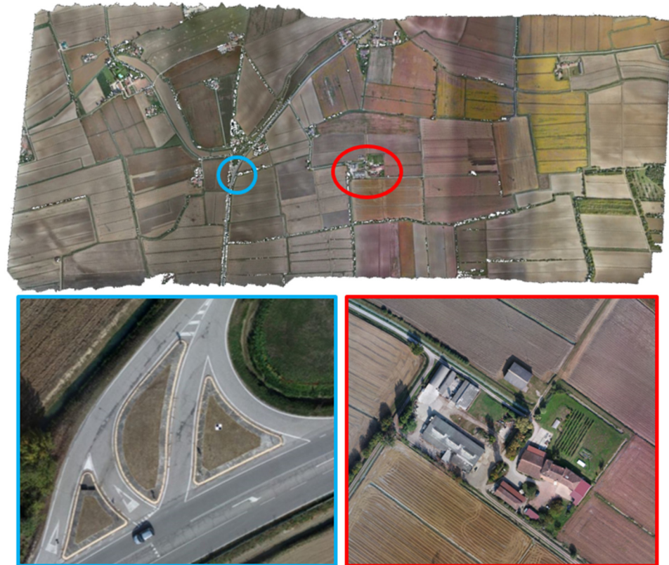
Figure 9. Ortophoto of the entire area obtained with Agisoft Metashape: simulation of a fast investigation of the overall situation of portions of the affected area surveyed during EXE 2.
