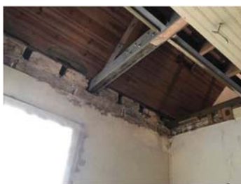
Figure 7 – Jointing the wooden beams and locking the masonry walls out of plane by connecting to the floor structure (credits: Aníbal Costa)
