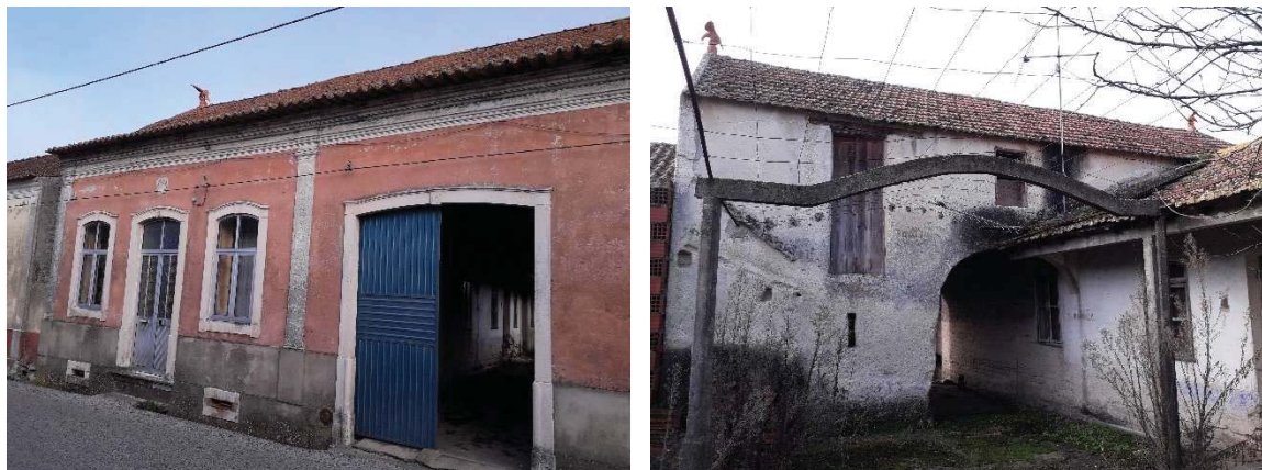
Figure 11 – Front facade and interior view of the courtyard of Gandaresa House, Seixo, Mira (credits: Aníbal Costa)
