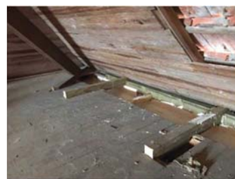
Figure 9 – Splice of wooden beams (credits: Aníbal Costa)
