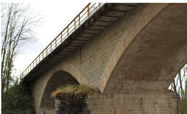
Figure 1. Views of Toppoli Bridge
