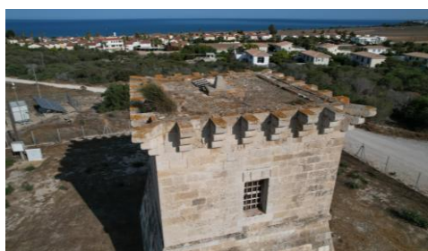
Fig. 1- View of the Tower in the landscape
