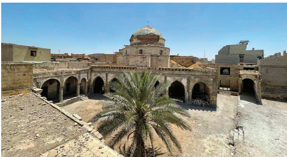
Figure 3: View of the mosque area taken from the rooftops of the madrasa before the start of architectural survey activities.
